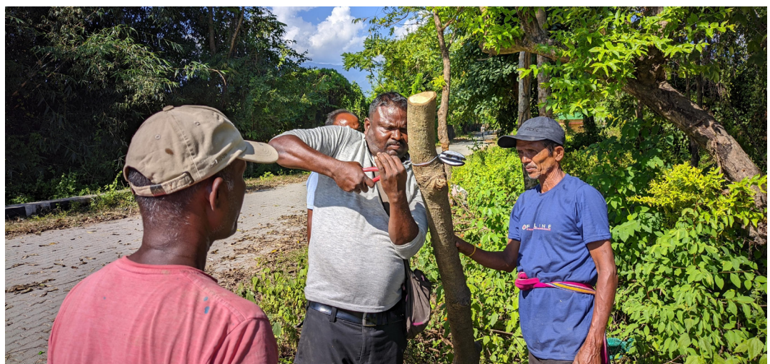
Solar fence installation underway in Udalguri district
