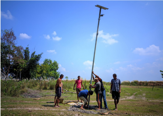
Solar street light installation in Goalpara district
