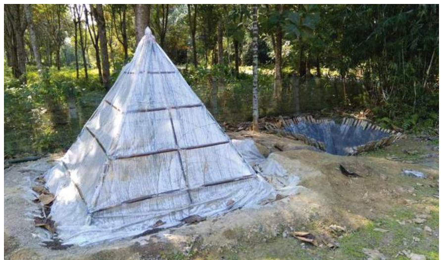
Polydome based rain water harvesting system installed at 2 No. Chourang Village, Panbari
