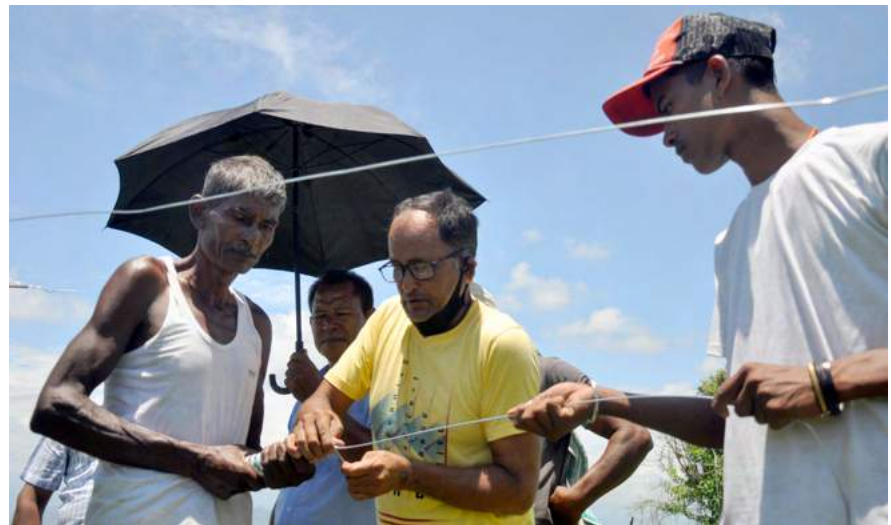
Installation of solar-powered fence
