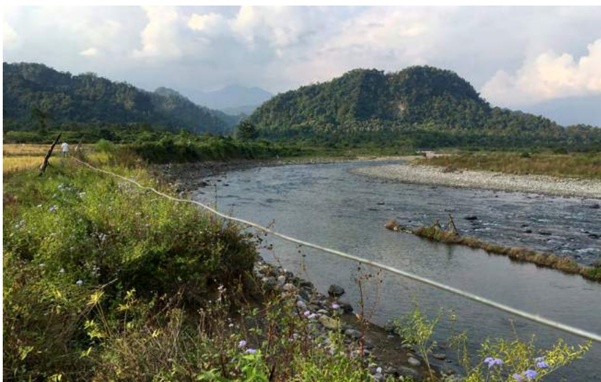
An illegal fence installed by local communities
