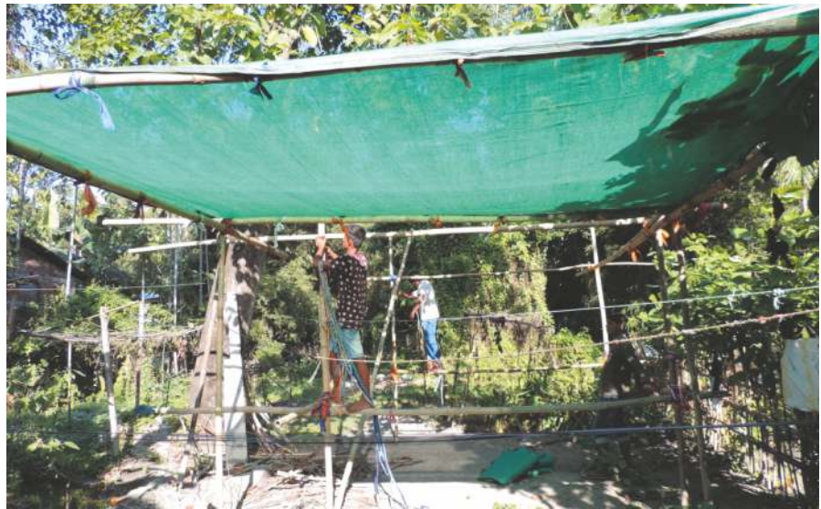
Net fitted under tree
