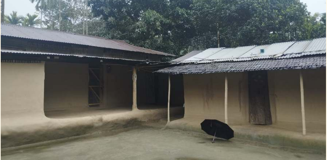
Traditional Adivasi house in Daodhara village
