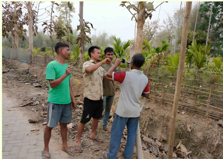
Community members working together to install a solar-powered fence
